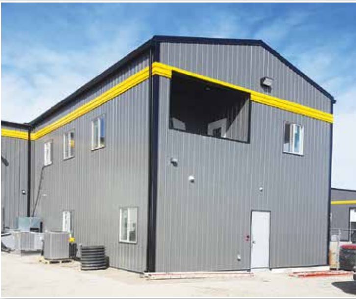
Dennis Dirtworx office addition Nitro Construction Ltd.
