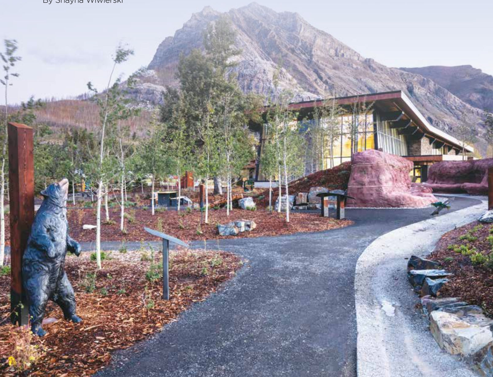
The new Waterton Lakes Visitor Centre is located in the middle of the Waterton townsite and will be open year round. PHOTO BY GRAHAM CONSTRUCTION.
