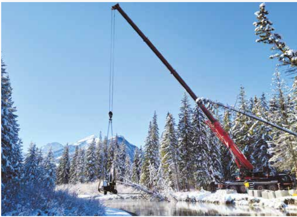
Syncline Barnaby Trail and Bridge deGraaf Excavating
