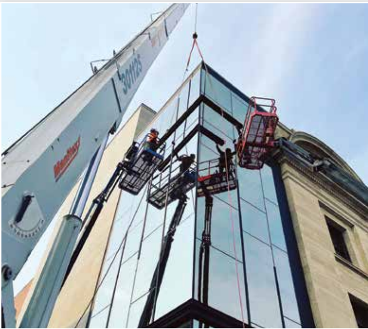
Post Office renovation Zero Gravity Crane & Rigging Inc.
