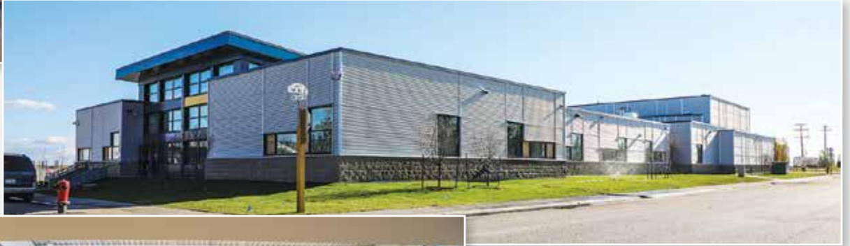
Tilley School Ward Bros. Construction
