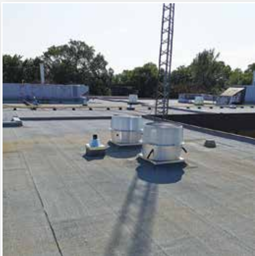
AHS Claresholm Roof Replacement Nitro Construction Ltd.
